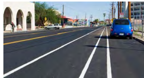
Bicycle Lane right-hand side buffer, Tucson, AZ
