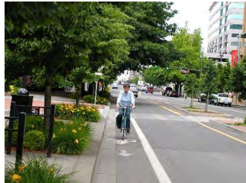
Bicycle Lane, Vancouver, WA
