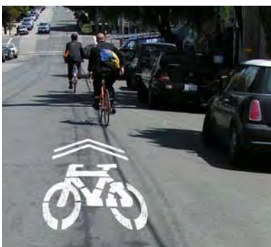
Shared Lane Marking, San Francisco, CA
