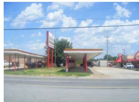
Existing Conditions: Lack of Sidewalks
