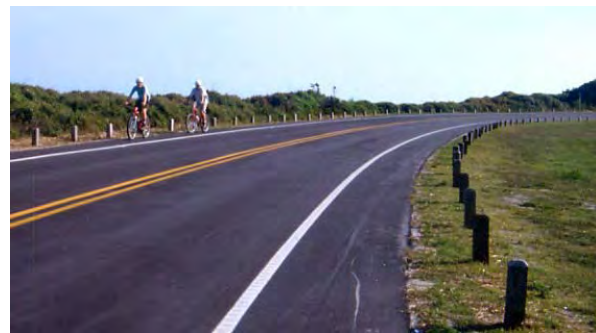
Paved Shoulder, Florida
